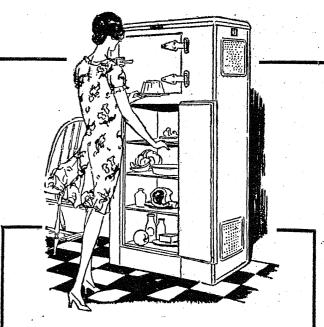
AS operates the Electrolux refrigerator. A tiny gas flame and a little stream of water start the refrigerating chemical on its endless cycle. The gas refrigerator is vibrationless and noiseless, and has no moving parts to wear out or to require replacement.
